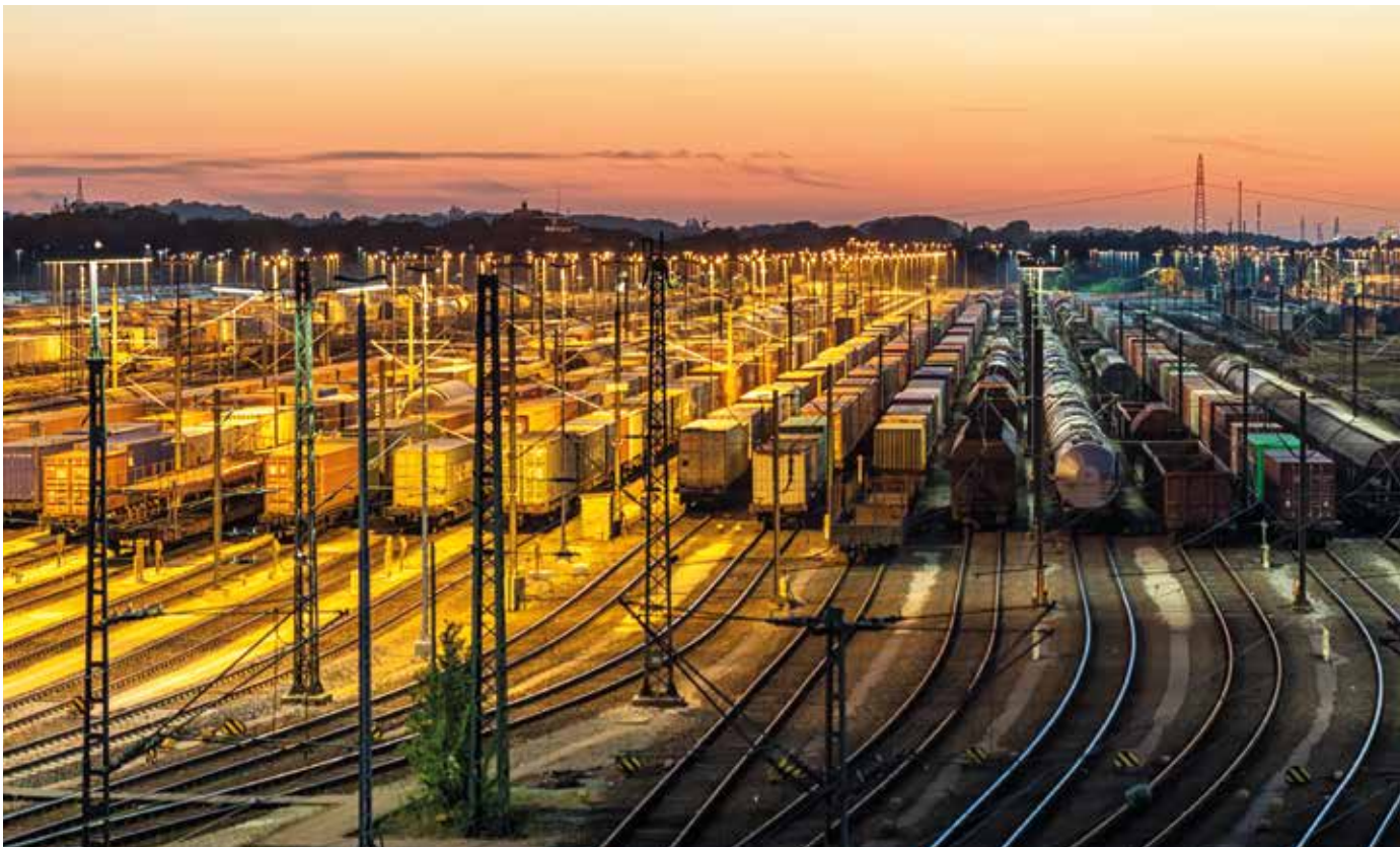
↑ Inductive wheel sensors are used for various applications in hump yards.
