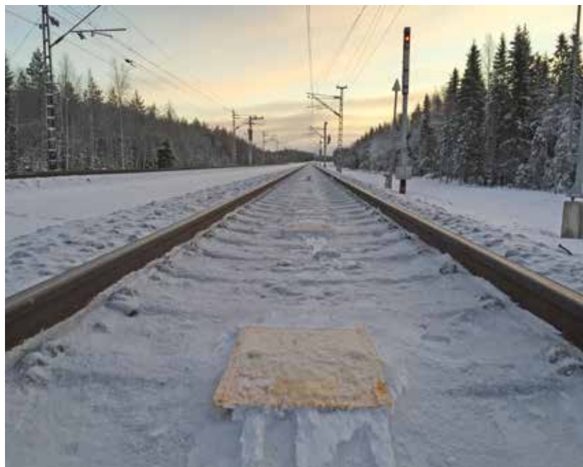
↑ Balises transmit information to passing trains.
