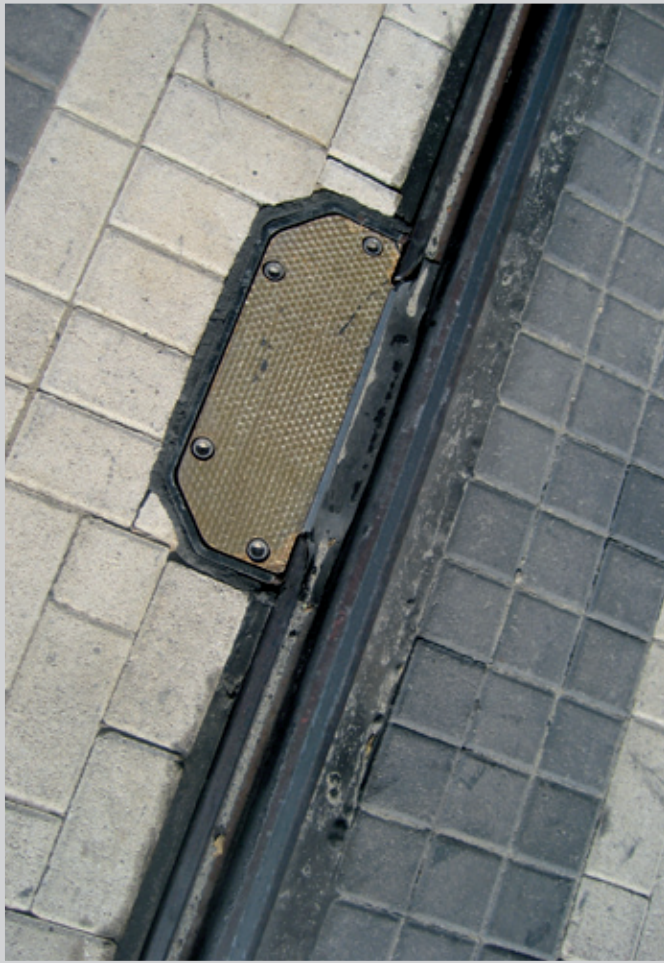
Figure 5: Robust and compact housing of the wheel detection components
