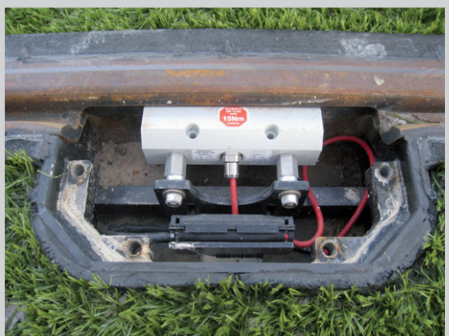
Figure 8: Compact arrangement and simple calibration of the wheel sensor due to Frauscher grooved rail claws
