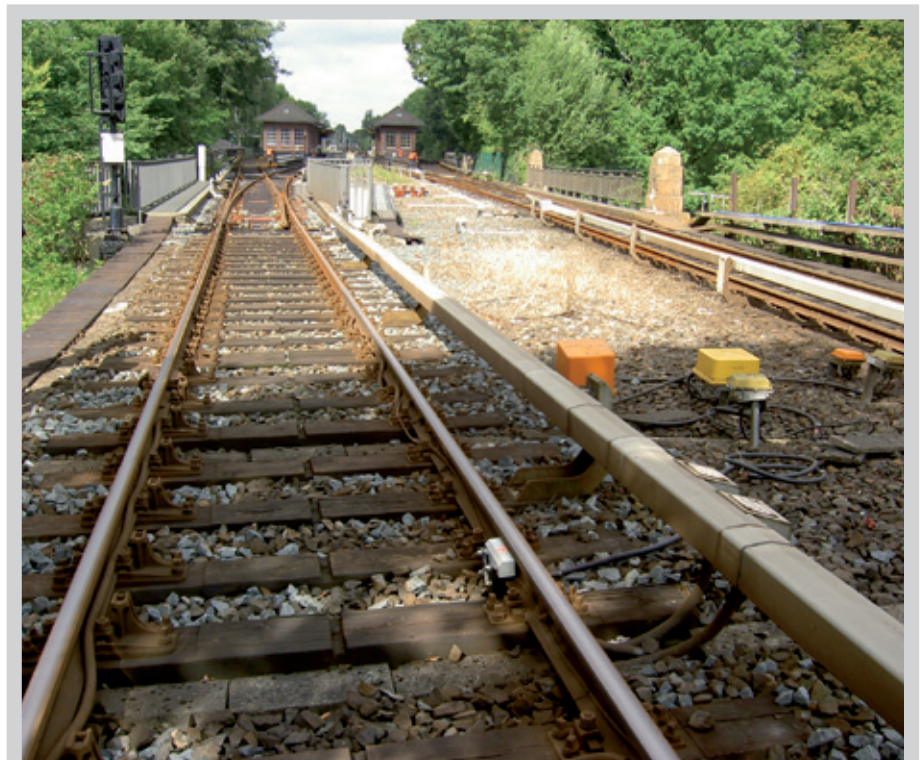
Figure 4: Wheel sensors must be resistant to direct current tractions
